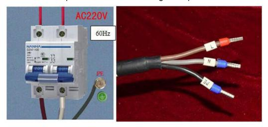
Note: This device is a large current equipment, with high requirements for the joint processing of power lines. Need compress the end of the power line directly and connect it to the wire holder of the air circuit breaker, and screw the bolt. Ensure to compress the power line end, no loose, otherwise will lead to accident or danger due to the heating caused by too large resistance at the thread juncture.
